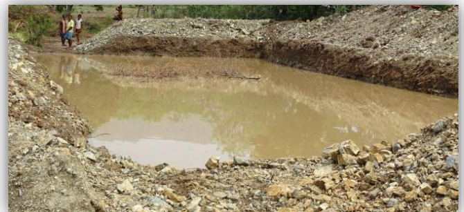
Rain water storage structure (20 ft x 20 ft x 5ft).
